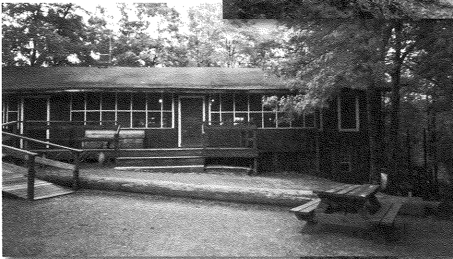
Jones recreation Hall Old Dining Hall
